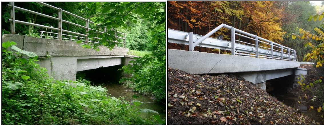
Figure 2 Stupava bridge before reconstruction and after reconstruction
