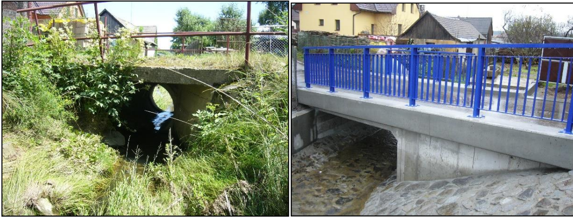
Figure 1 Kozlov bridge before reconstruction and after reconstruction
