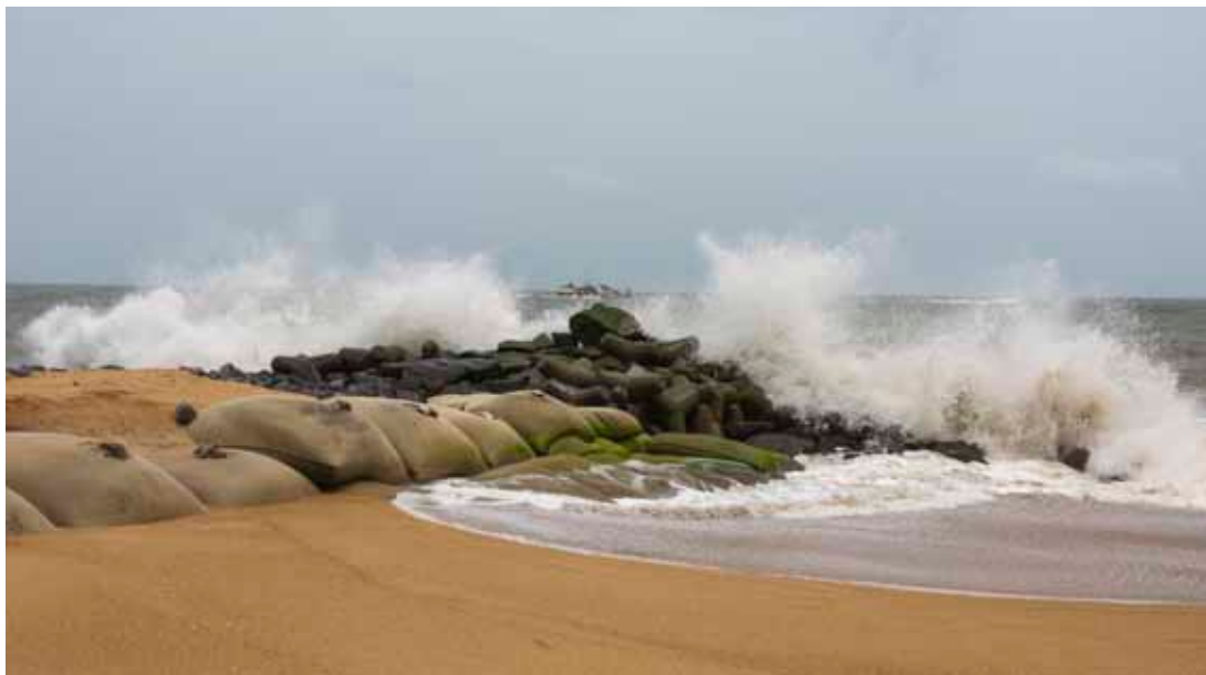
Beach protection. Construction of berms under the Sustainable Coastal Protection and Management Investment Program, Ullal, Karnataka, has reclaimed the beach and protected the assets of fishing communities (photo by ADB).
