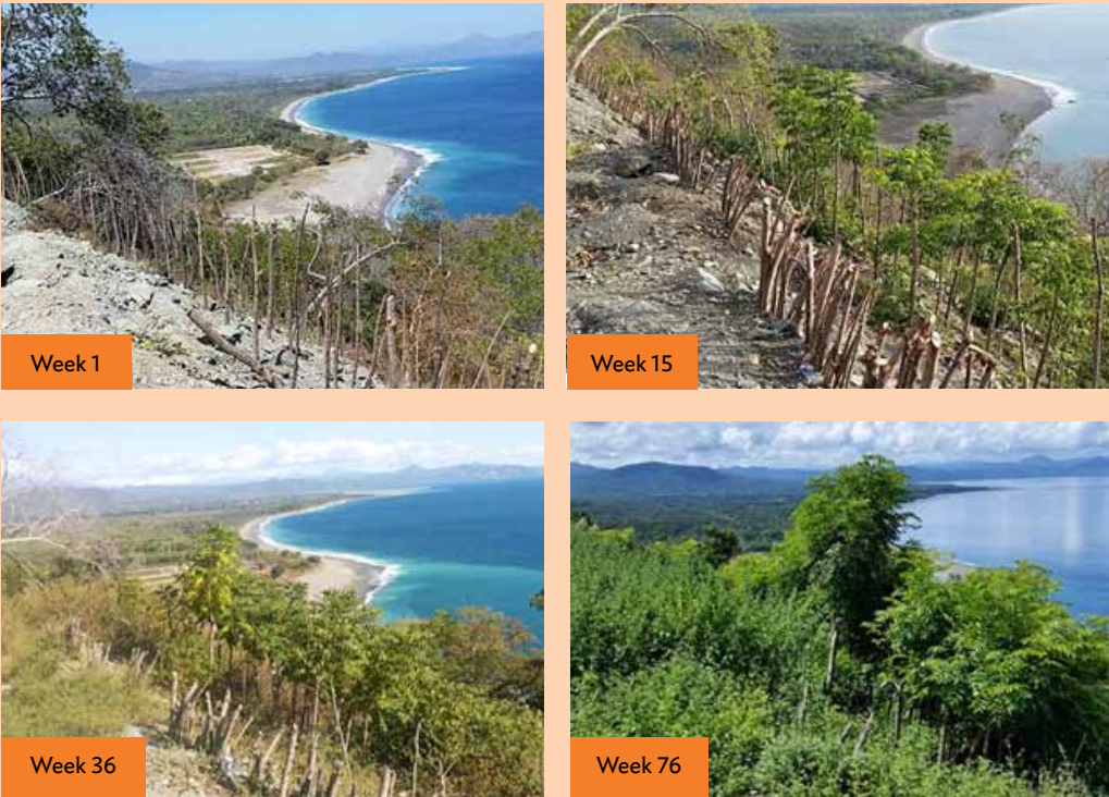
Figure 3: Using Live Stakes Method in Soil Bioengineering
