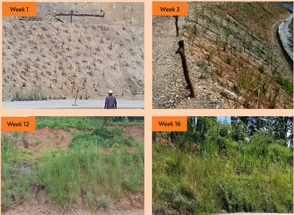
Figure 4: Using Mixed Grasses in Soil Bioengineering
