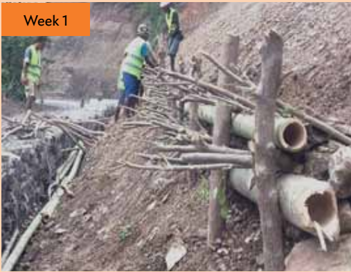
Figure 5: Using Rock- and Vegetation-Based Reinforcement in Soil Bioengineering
