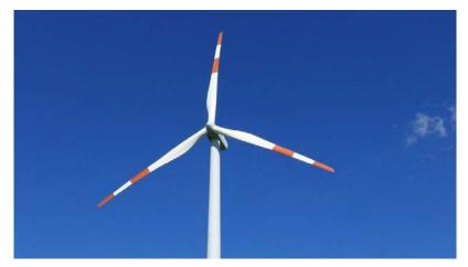
Figure 5.3 Initial position of blades prepared for inspection [5]
