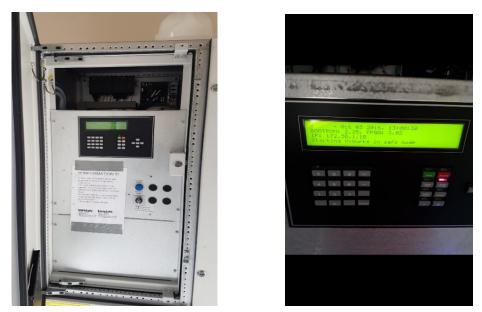
Figure 5.2 PLC control module (SCADA interface)
