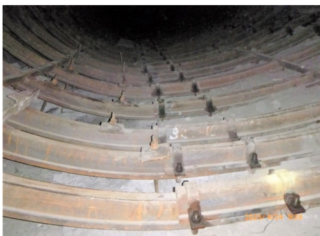
Fig. 12. Horseshoe-shaped reverse vault and anchors before concreting
