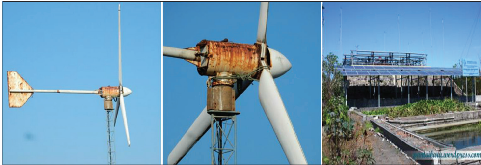
Figure 2: Corrosion in wind turbine and PLTH system
