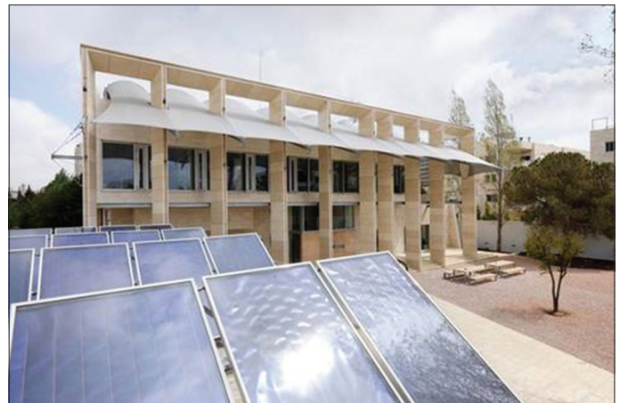
Figure 4: Solar thermal panels for hot water in the garden of the embassy
