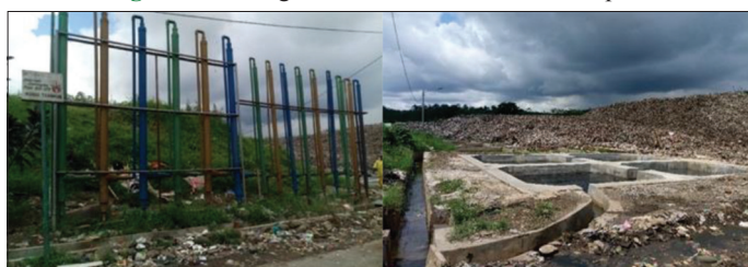
Figure 5: Flaring and leachate water treatment pool
