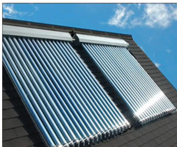
Figure 2: Evacuated tube collectors
